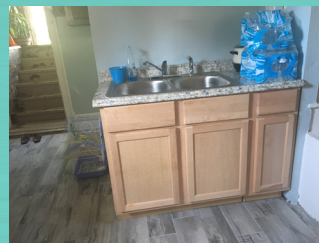
Cervantes Family's kitchen after repairs
